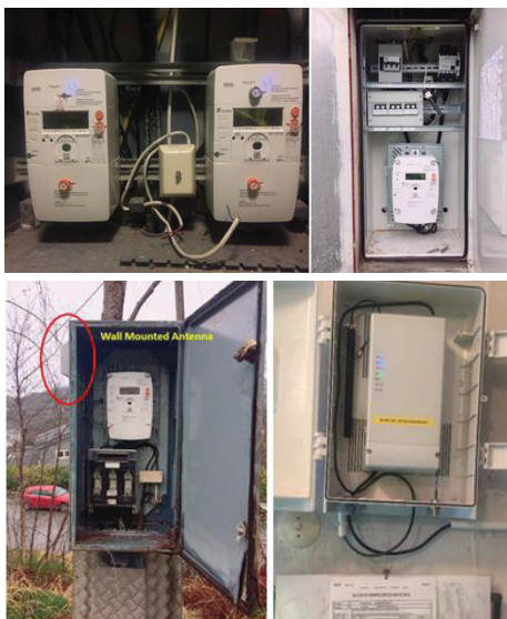
Security DCU and smart meter applied with commercial AMI (250,000 households in Bergen, February, 2018)
